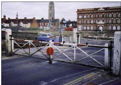
Existing manned mechanical gate crossings at Boston, Lincolnshire
